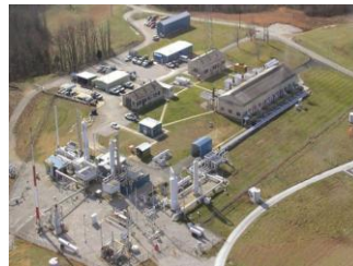
NG Compressor Station
