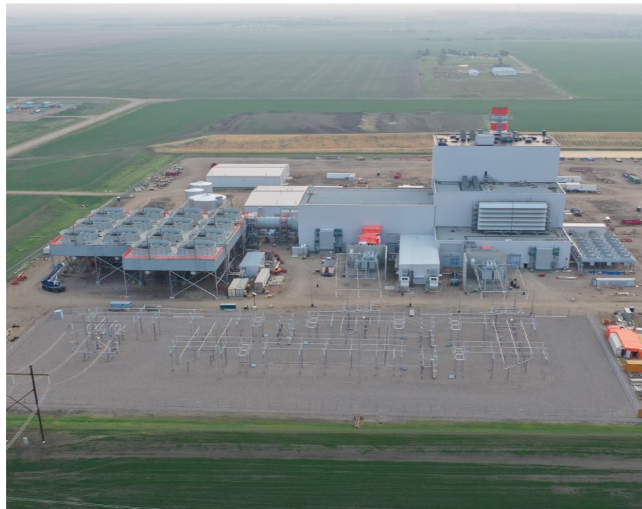
Great Plains Power Station - under construction
