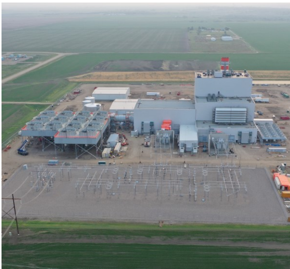
Great Plains Power Station - under construction
